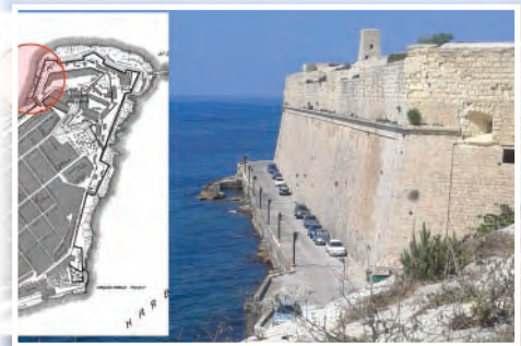
Fig. 02 Saint Gregory's Bastion, Valletta. The foreshore was encased in concrete in the early 1980s. Inset: Detail from 1927 Survey Sheet published by the Office of Public Works, Valletta, showing position of bastion and configuration of shoreline prior to casting of concrete.
