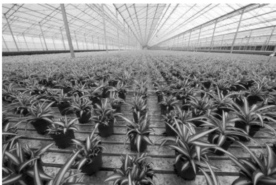
Figure 20: Detail of the interior of the photovoltaic greenhouse farm “Su Scioffu”
