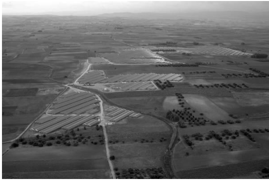
Figure 18: The photovoltaic greenhouse farm “Su Scioffu”
