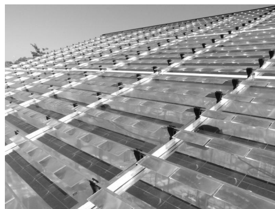
Figure 17: The prototype of photovoltaic greenhouse of Bizkaia
