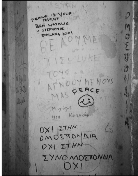
Figure 27 Graffiti on Guttered Buildings by the 'Dead Zone'. Text says: 'We want our Missing back'.
