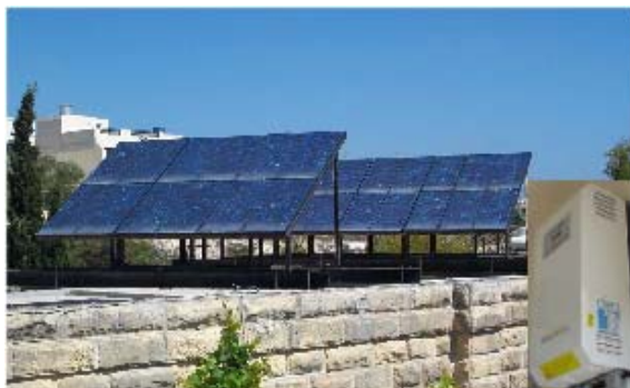
Figure 3: The Institute's 1.8 kWp grid-tied solar photovoltaic system with the inverter shown to the right.
