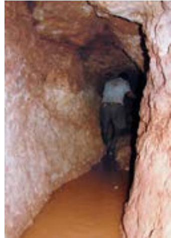
Fig. 7: Interior view of a perched aquifer gallery at Wied Ħażrun. In the Cabreo Antico della Procura delle Distribuzioni of 1621, this is indicated as a fontana or fountain (Source: the author)
