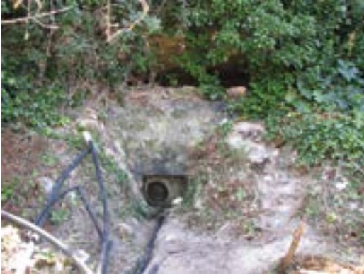
Fig. 13: The exterior of the fontana mentioned in NLM, Treas. B. 289, f. 84. Its location is indicated on a plan of the Tal-Callus estate in NLM, Treas. B. 291, f. 86. This water source originates from a perched aquifer gallery which is fronted by a subterranean water storage reservoir. A series of steps to the right of the water sump facilitates access to the reservoir interior. (Source: the author)
