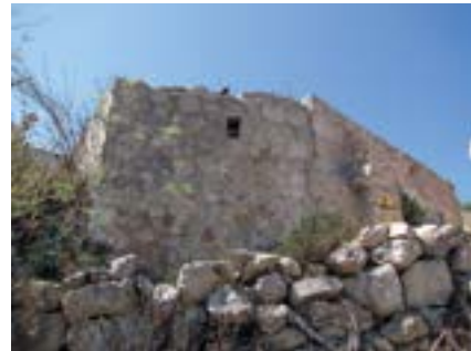
Fig. 16: The Tal-Callus estate hamlet at Wied ir-Rum. Exterior view of the probable Late Medieval church dedicated to either St Nicholas or Santa Marija. What appears to have survived of the original church fabric betrays the presence of a gabled ceiling, and a narrow slit-like window is located high up in the north façade of the structure (Source: the author)
