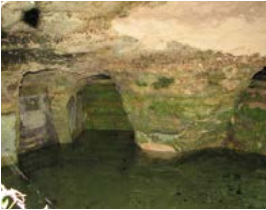
Fig. 14: Interior view of the fontana mentioned in NLM, Treas. B. 289, f. 84, the location of which is indicated on a plan of the Tal-Callus estate in NLM, Treas. B. 291, f. 86. This water source originates from a series of galleries, a number of which were walled up at an unknown date. The extracted water is stored in a fronting subterranean reservoir (Source: the author)
