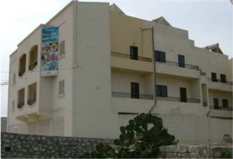
Figure 1a: Photograph of the Northern and Western elevations.
