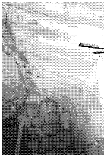
Fig. 5 Cave dug into the west face of the Il-Qlejgha tal-Bahrija promontory in the territory to Bahrija, Malta. Detail of mortar rendering covering the ashlar slabs bridging the gap between the screening wall and the overhanging rock-face.
