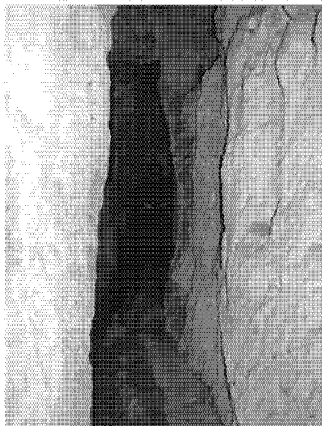
Fig. 15 Interior view of a rock-excavated water gallery, tapping a ground water source in the territory of Ferla, Sicily.
