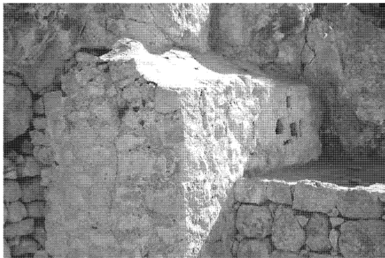
Fig. 6 Ashlar slabs bridging the gap between the screening dry-stone wall and the overhanging cave-roof at Gnien San Gakbu settlement in the territory of Rabat, Malta.
