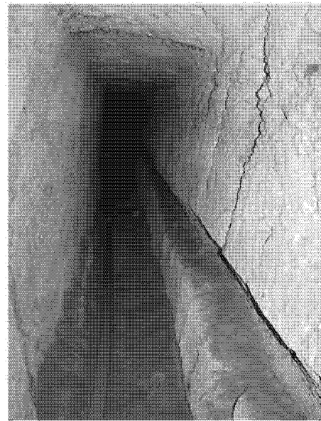
Fig. 14 Interior view of a rock-cut, perched aquifer water gallery at Tas-Santi in the territory Mgarr, Malta.
