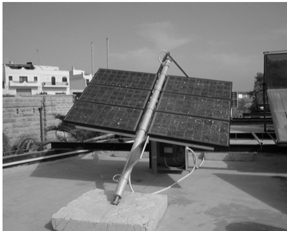
Figure 3: A solar array of 6 modules attached to a tracking mechanism, which is being driven by an inbuilt dc motor operated by a bi-facial solar module.
