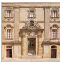
Cover: During the 1837 cholera epidemic Vilhena Palace in Mdina served as a temporary hospital. In 1860 it was used as a sanatorium for British troops. Early in the 20th century the palace was passed to the Maltese government and was converted into a hospital for tuberculosis patients and was formally inaugurated by King Edward VII on 22 April 1909 and was referred to as the Connaught Hospital. On 10 January 1956 the hospital closed down. Today the building houses the National Museum of Natural History. - Heritage Malta
