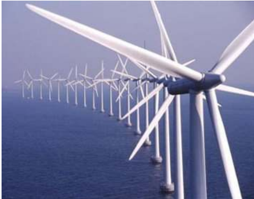
Figure 8: Offshore wind farm in Danish waters.
