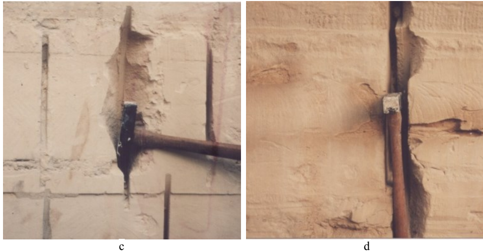
Fig. 1 (continued) – Lower Globigerina Limestone (a) with burrowing (b) iron stained burrow infill (c) and weathering of burrow infill (d). For scale purposes, the head of the geological hammer is 160 mm long.
