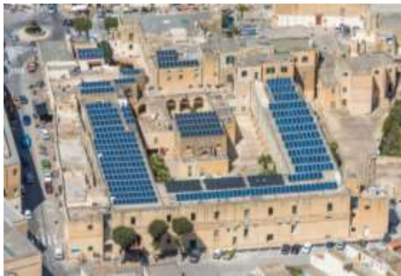
Figure 1: The Ministry for Gozo Administration Centre
