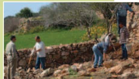
March 2004. Rebuilding rubble walls.
