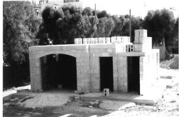
Workshop, store and office compound taking shape at Is-Simar.
