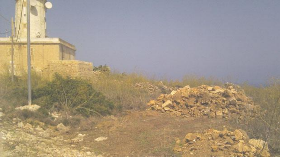
Mounds of rubble dumped near the Tal-Ġordan lighthouse, Ghasri, by a contractor engaged to repair the approach road to the lighthouse.
