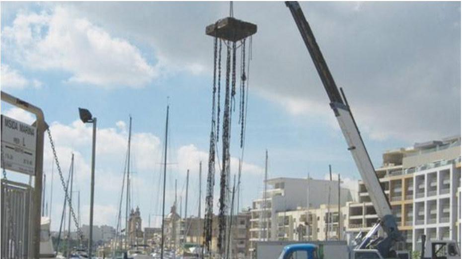
Mepa forced a contractor entrusted to revamp the Ta' Xbiex yacht marina to recover hundreds of tons of rusted chains from the seabed at Ta' Xbiex and Msida.
