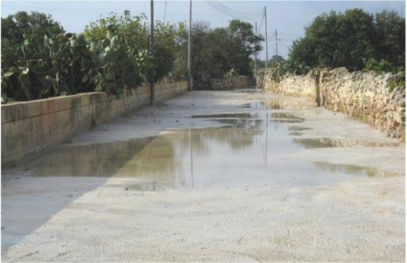
Short-sighted action has concreted over a former groundwater recharge zone, leading to flooding.
