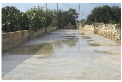
Short-sighted action has concreted over a former groundwater recharge zone, leading to flooding.
