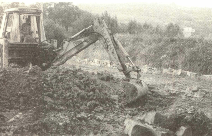
Scratching the surface. A small JCB excavates the initial foundation hole.
