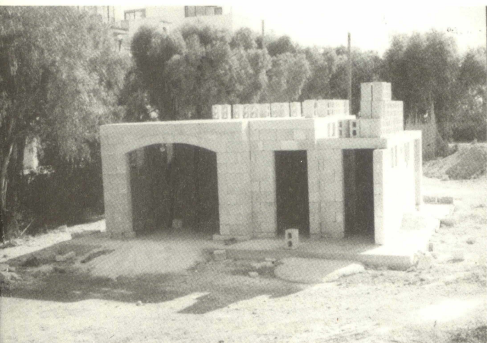
Shell complete. The building will incorporate workshop, store and toilet/shower facility.
