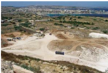
The waste disposal facilities at Maghtab.
