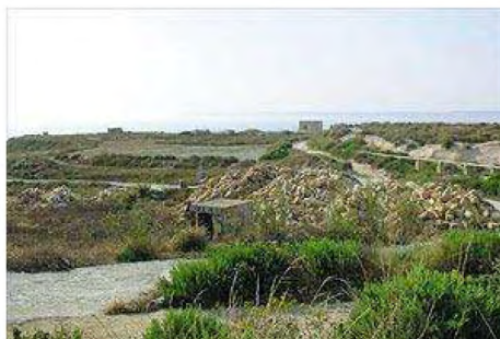
The dumping of building debris further downhill at Bahrija
