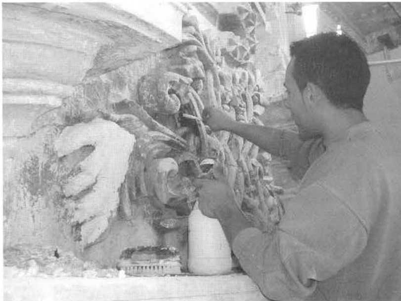
Here and above: Restoration work at Sarria church
