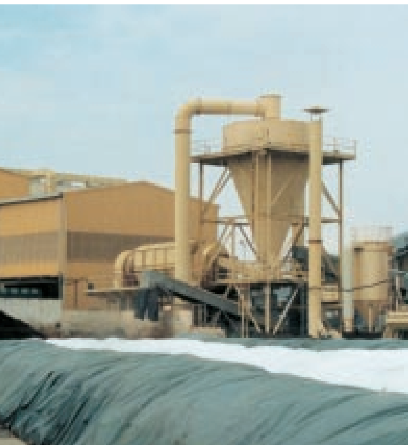
The Sant' Antnin Waste Treatment Plant
