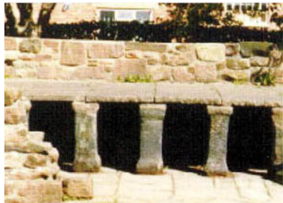
Figure 1: raised floor on stump walls with gaping openings for cross-ventilation
