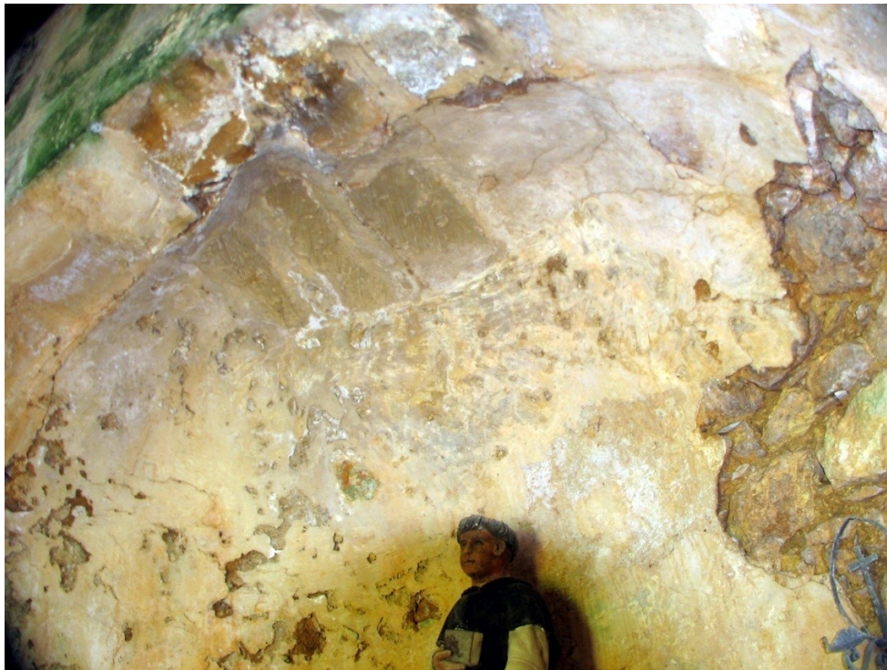
Plate 7 Roof slabs bridging the gap between the keystone section of the arch and the adjoining wet-rubble wall.
