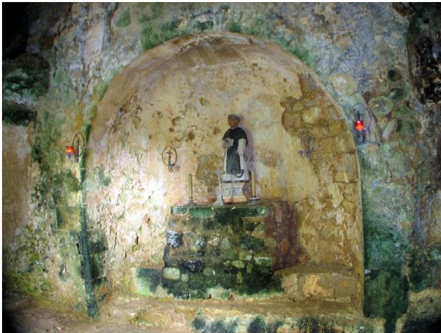
Plate 4 St Leonard cave-church. East-end cylindrical apse and altar built partly of ashlars and wet-rubble.
