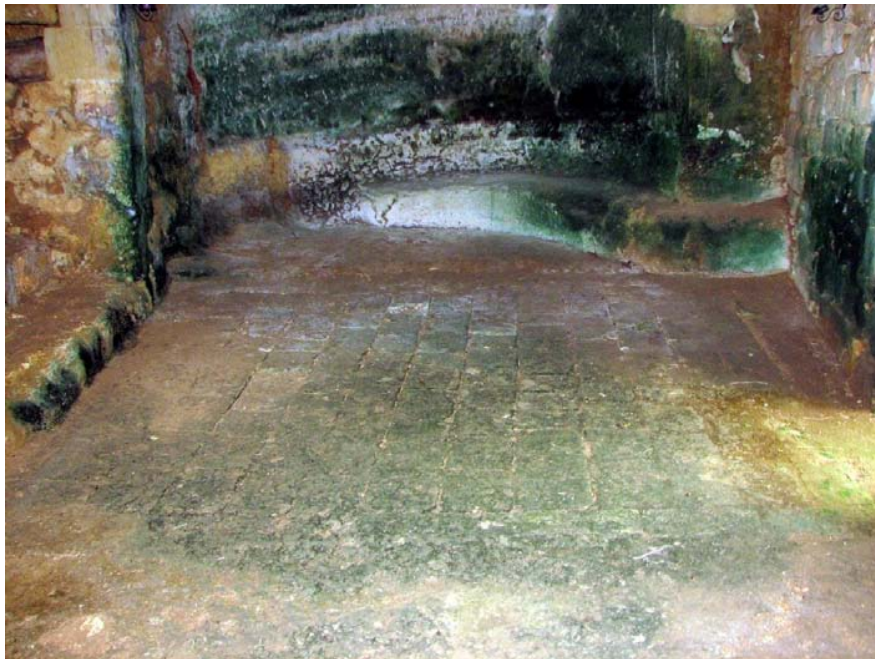
Plate 17 Flagstone floor detail. Visible in the foreground is the rock-cut bench (dukkien).
