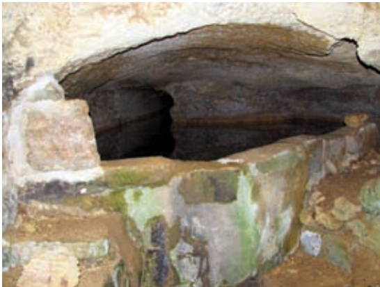
Fig. 10.7. Underground water reservoir fronting gallery entrance in Wied Liemu l/o Rabat.
