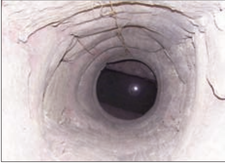
Fig. 10.9. Vertical shaft at Palazzo Falsone, Mdina, giving access to a probably underlying water gallery.
