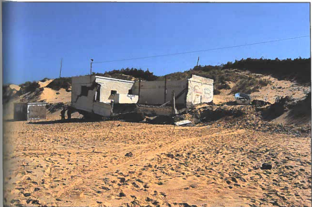
Plate 38: Collapse of coastal constructions following extensive beach erosion at Zouaraa, Tunisia
