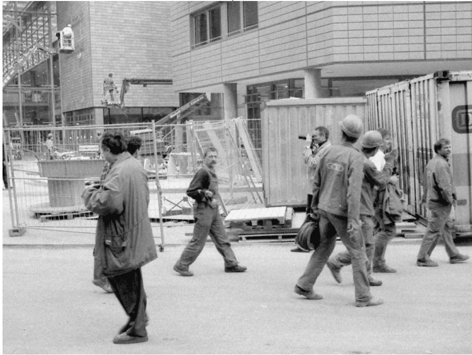
Construction site, Potsdamerplatz, 1998. To the amusement of workers, tourists snapped up one photo opportunity after another as they idled through Potsdamer Platz.
