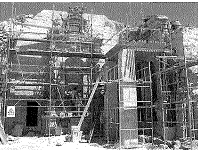
Plate 3. Erecting the scaffolding
