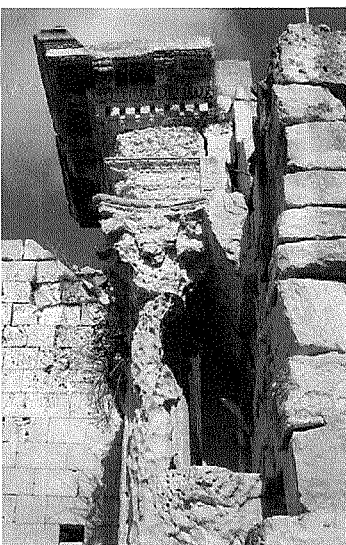
Plate 4. A highly eroded column and architrave
