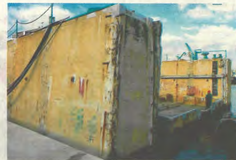
One of S. Bezzina's reinforced concrete floating docks.
