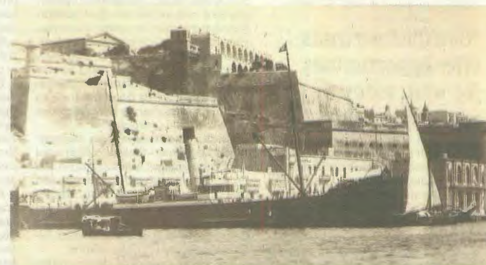
The Barrakka Lifts saved the ferry company additional investment.
