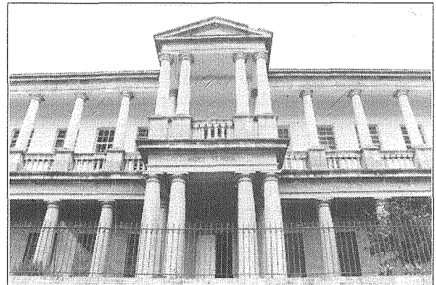
Żejtun Primary School, detail of façade
