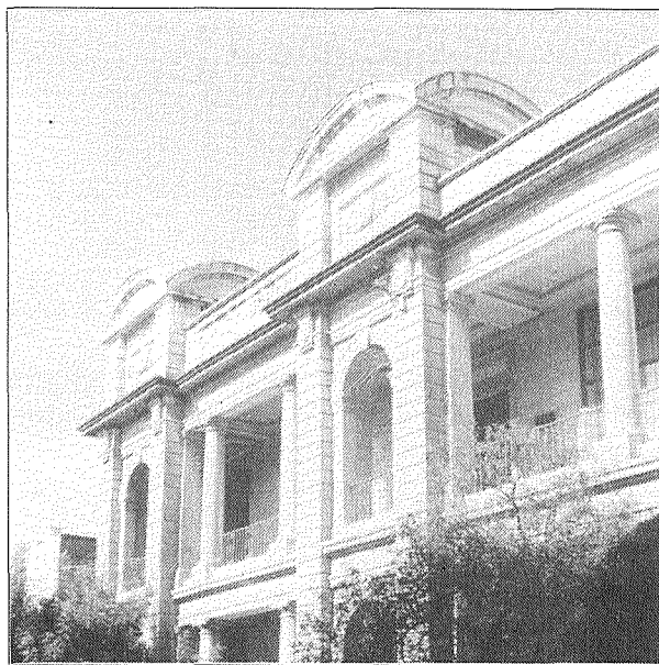
Sliema Primary School, detail of facade
