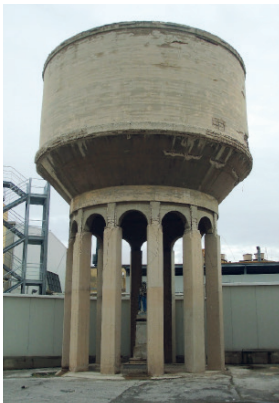
Figure 1a. Reinforced Concrete Water Tower, Public Abattoir, Marsa, Malta.
