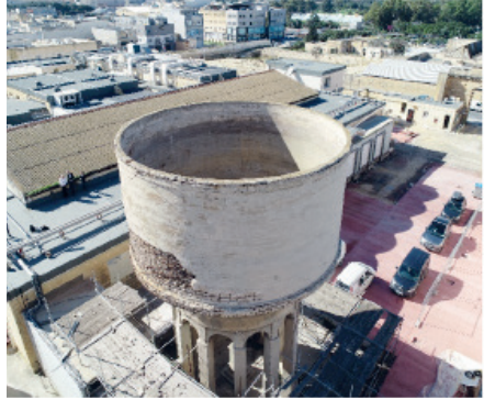
Figure 1c. Aerial view of the water tower.
