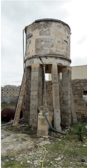
Figure 3a. Water Tower at the Gzira Pumping Station, Malta.
