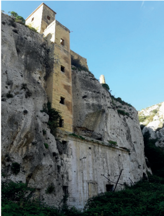
Figure 4a. The Mġarr ix-Xini pumping Station.
