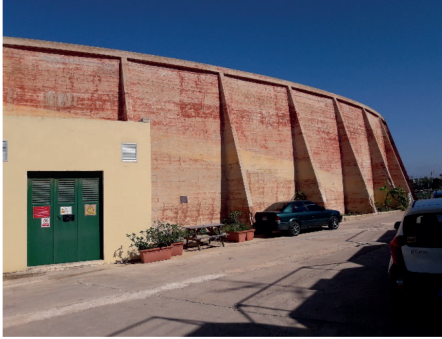
Figure 7a. The Maghtab Acoustic Mirror buttressed structure from the back (2017).
