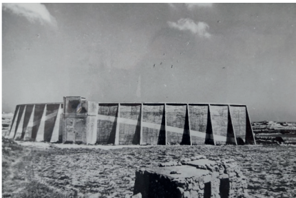
Figure 6a. The Magħtab Acoustic Mirror buttressed structure from the back.
