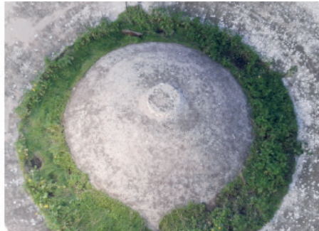
Figure 2b. The interior of the tank.
