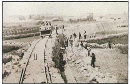
railway embankment is being encased with masonry in 1882
