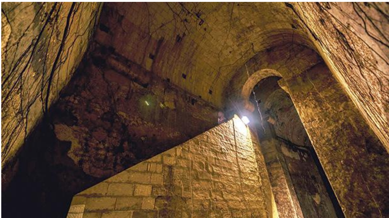
View of one of the cisterns.
