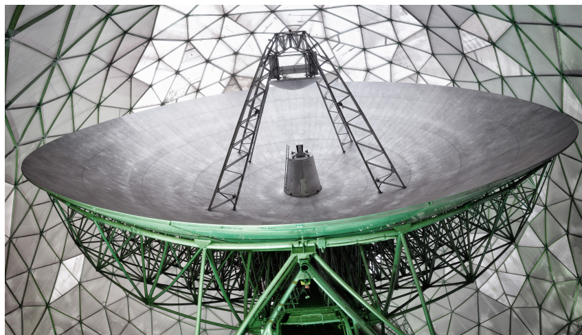
Figure 1.9: The 34 m diameter parabolic reflector at the TIRA radar facility in Wachtberg, Germany (Source: Fraunhofer Institute for High Frequency Physics and Radar Techniques (FHR))
