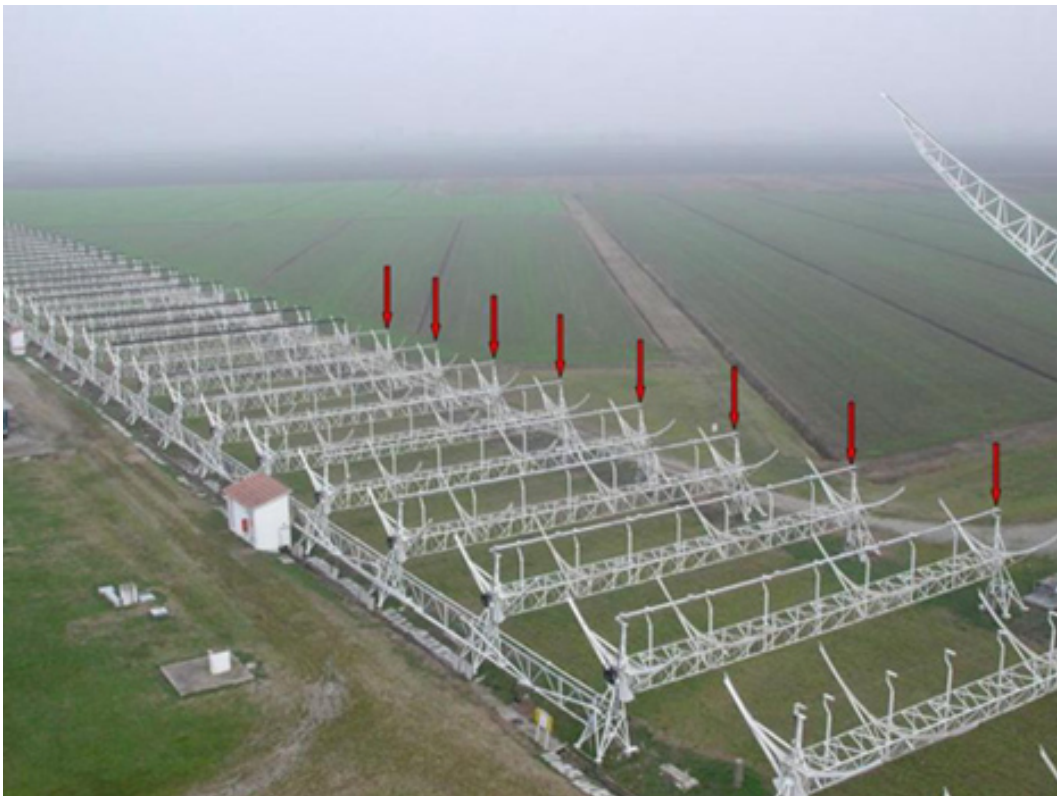
Figure 2.2: The eight East-West cylindrical concentrators making up the BEST-2 array within the Northern Cross. Source: www.med.ira.inaf.it
