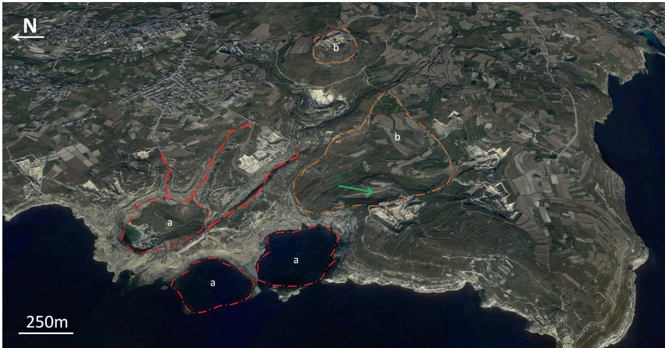
Figure 1.5. Characteristic geomorphological features developed on the Lower Coralline Limestone in western Gozo (Dwerja Point). The picture shows different sub-circular collapsed karstic features (a & b), while the green arrow points to the location of the chert outcrops (image © 2017 Google).
