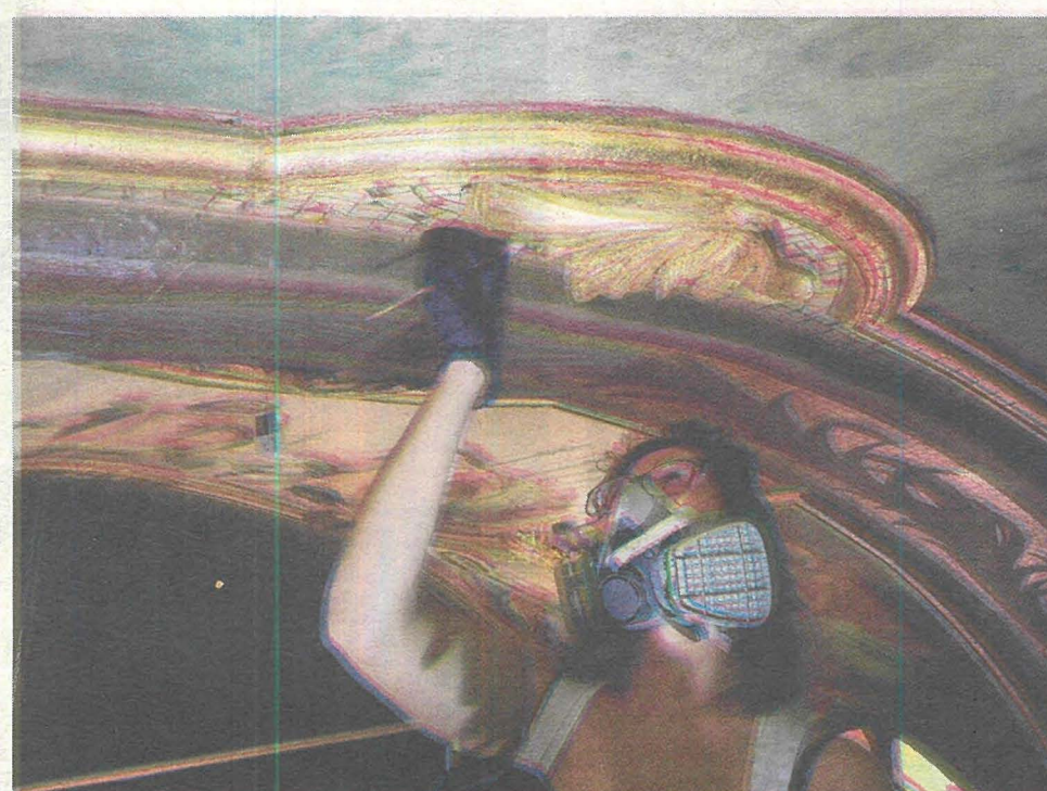
Cleaning of the gilded wooden decorative cornices.
