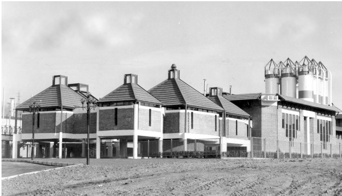
Figure 2. Bread Factory, Tbilisi: View as in 1980s (top), plan as built (bottom)
