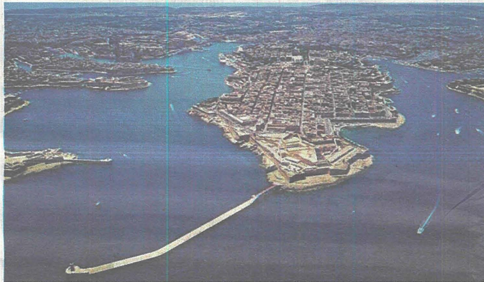
An aerial view of Grand Harbour showing the two arms of the breakwater.
