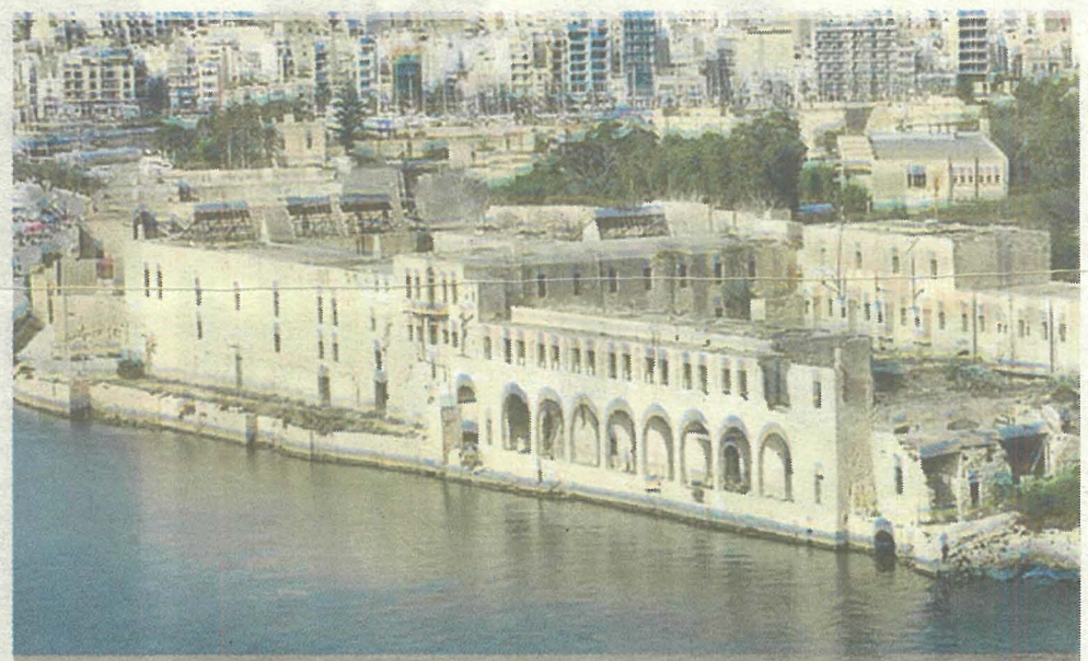
Lazzaretto Hospital at Manoel Island, now in a dilapidated state.
