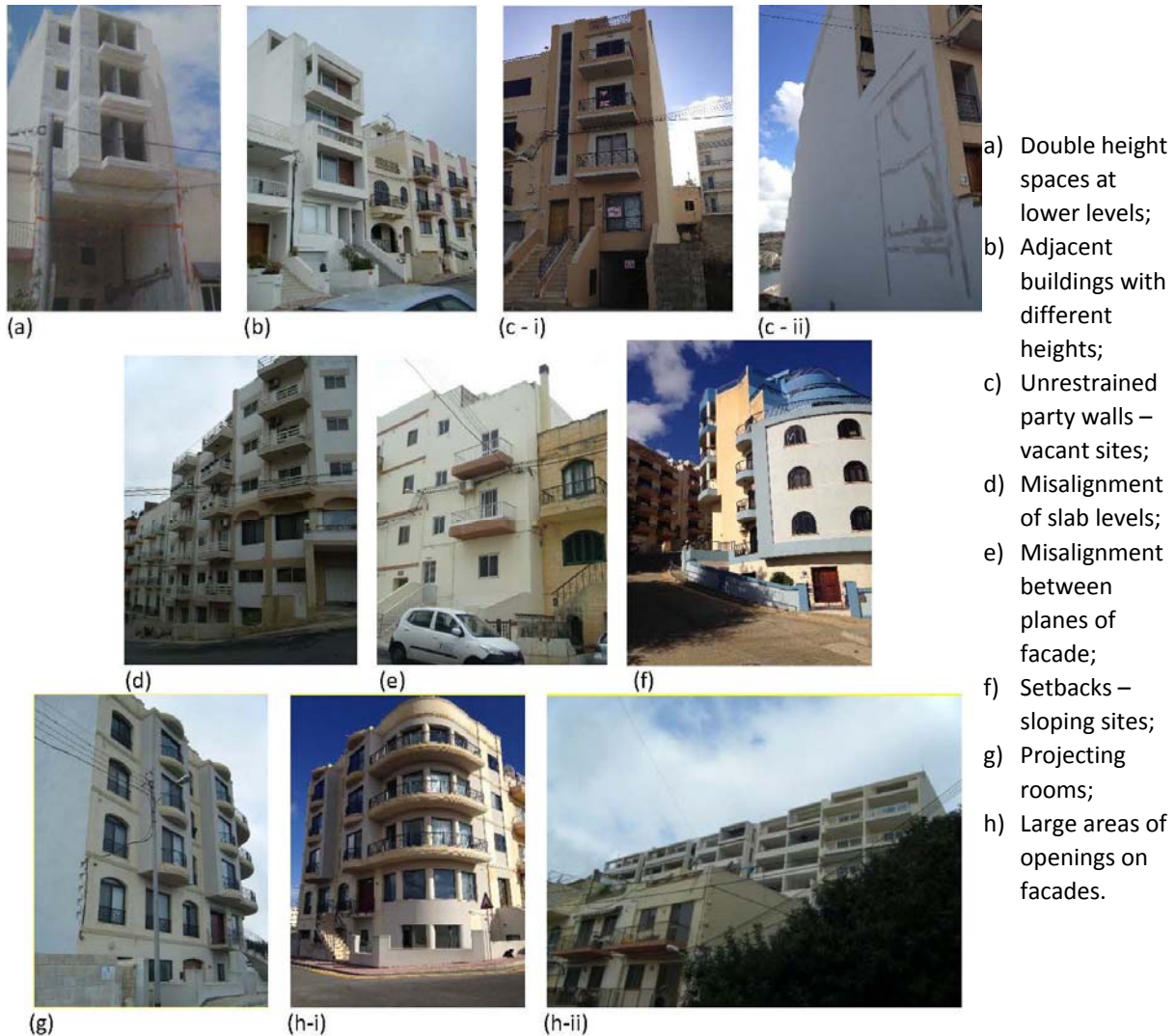
Figure 1-1 Examples of building characteristics commonly found in the contemporary loadbearing URM building typology and which could impair the seismic resistance of this construction typology ([5]p. 137, 138; [6] p.289).
