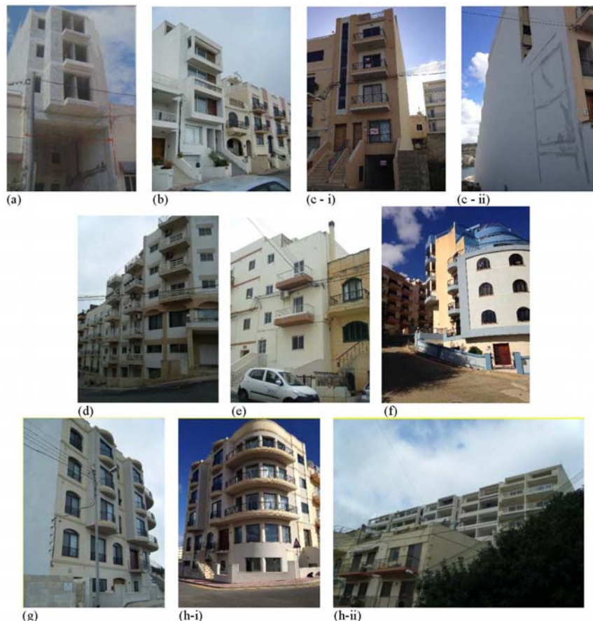
Figure 1: Examples of seismic vulnerability characteristics present in the contemporary loadbearing masonry building typology -1: (a) double height spaces at lower levels due to commercial establishments; (b) adjacent buildings with different heights: unrestrained party walls and misaligned slab levels; (c) unrestrained party walls due to vacant sites; (d) misalignment of slab levels within same individual buildings and between adjacent buildings; (e) misalignment between planes of facades of adjacent buildings; (f) setbacks – sloping sites; (g) projecting rooms; (h) large area of openings on façade.
