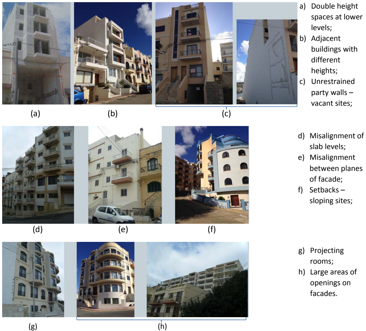
Figure 2: Examples of seismic vulnerability characteristics present in the contemporary loadbearing building typology present in the Maltese Islands (Torpiano et al. 2016).
