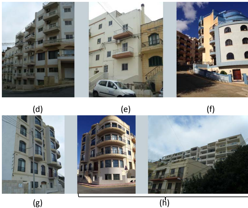
Figure 5b: Examples of seismic vulnerability characteristics present in the contemporary loadbearing masonry building typology - 2:
