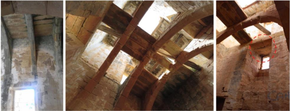
Fig. 12. Roof: (left) of entrance hall, (middle and right) of the first room to the right of the entrance with part of the collapsed roof of the first floor also visible; (right) failed masonry slabs are circled in red
