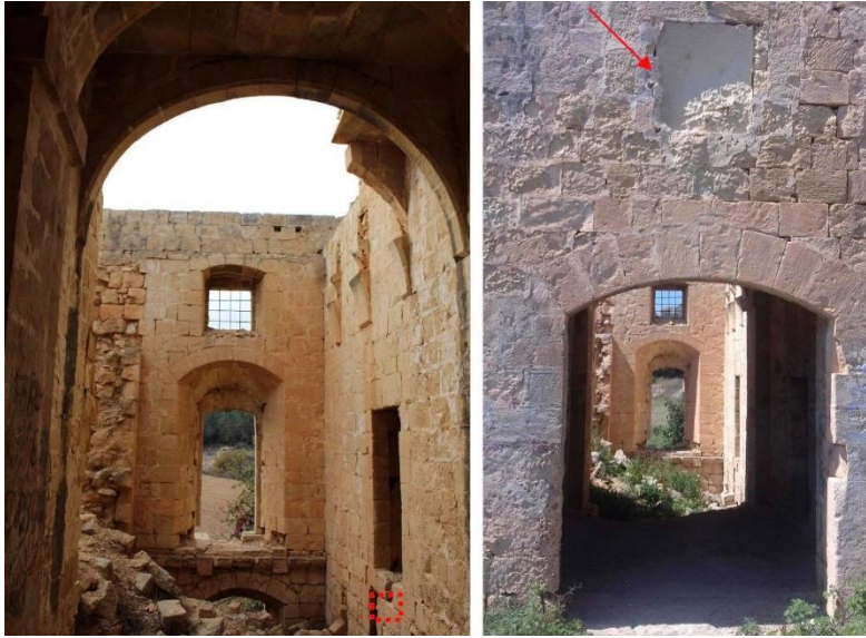
Fig. 13. (Left) the wall at the lower level erected in Coralline Limestone: detail indicated in red is shown in fig. 9 (left); (right) position of the inscription is indicated in red
