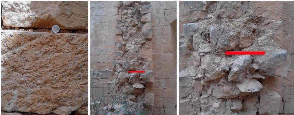
Fig. 9. (Left) damp-resistant layer of Coralline Limestone - for location of photo see fig. 13 (left); a €2 coin is used for scale, (middle) section through collapsed internal wall, and (right) detail of section; marker is 500 mm in length
