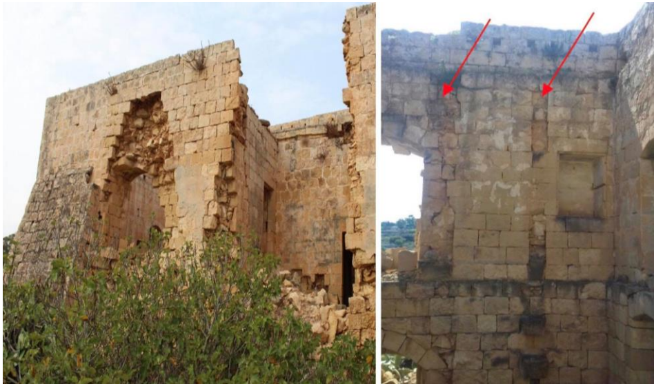
Fig. 10. (Right) the buttress on part of the southwest-facing elevation and (left) the position of the arches is indicated by a red marker
