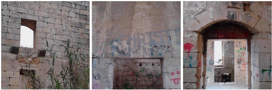
Fig. 11. Spanning openings over 0.9 m: (left) lintels with notched dimension stone, (middle) lintel depth increased from the standard 270 mm course height to 400 mm, and (right) arches introduced for spans over 1.1 m
