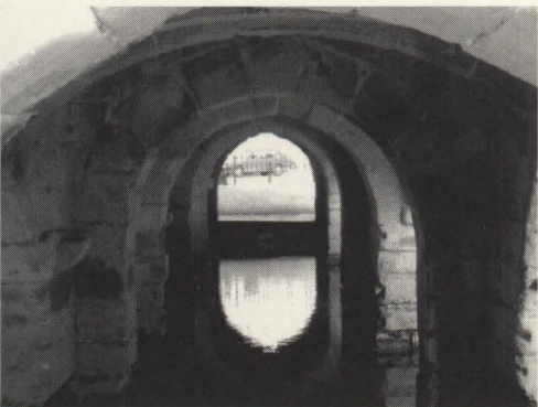
The interior of the wash house, which still contains water (Photo: Theresa Vann)
