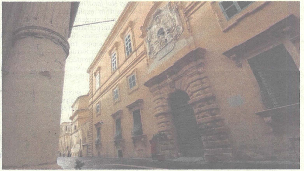
Main facade of Auberge d'Italie following restoration works on the main facade completed in August 2017.
