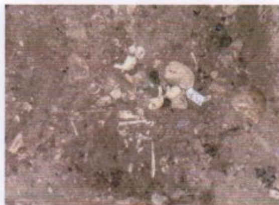
Figure 4: In-situ photograph ( En-Sure Monitoring image provided by the Superintendence of Cultural Heritage).
