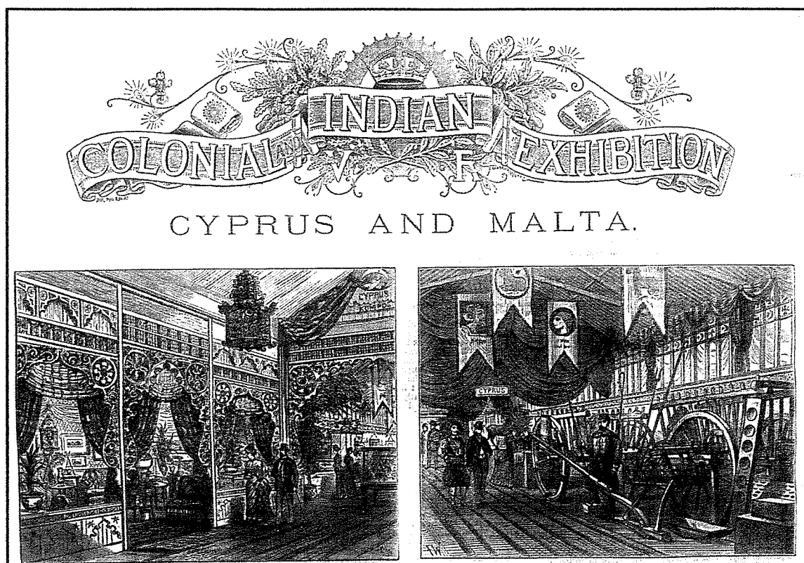
Fig. 2.11.11 (Left) North End of the Cyprus Court (Right) South End of the Malta Court (Source: Illustrated London News , October 1886)
