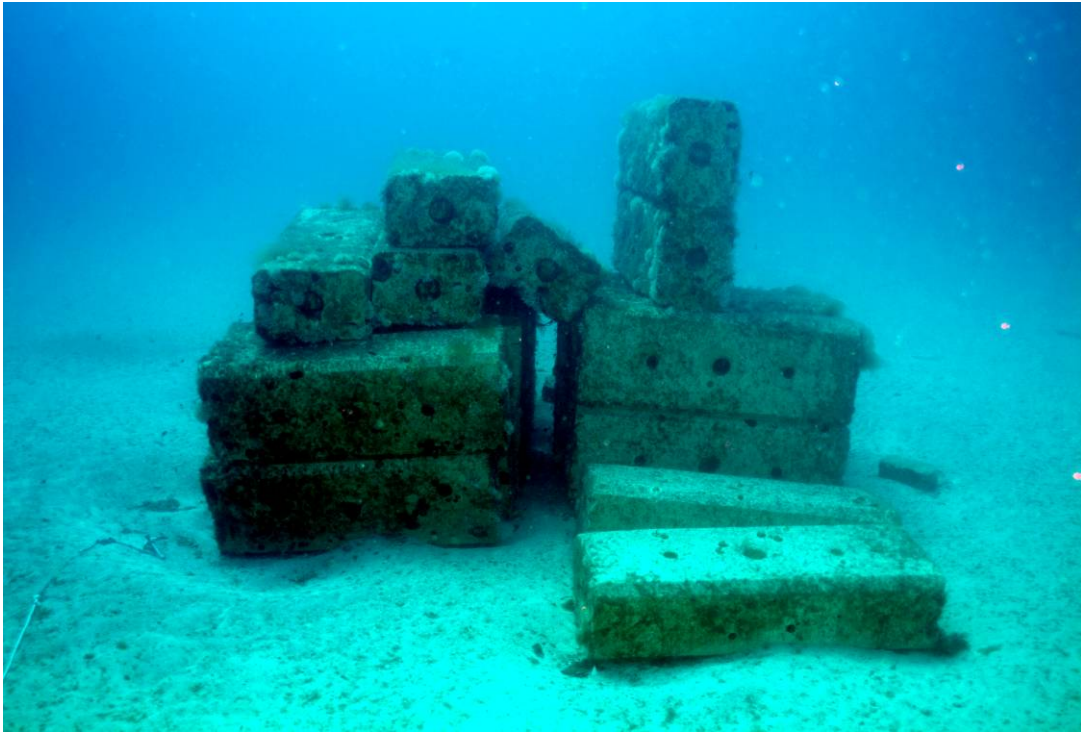
Figure 22. Photograph of the seabed and the artificial reef at Reef Area 2, showing hollows in the soft sediment (arrows) produced by scouring and collapse of some of the units. The photograph was taken in May 2005, eight months after deployment.
