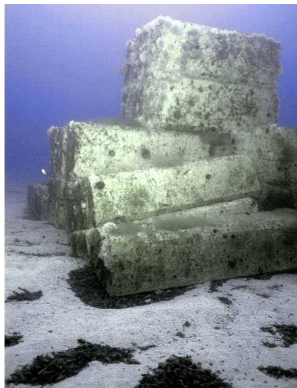
Figure 21. Photograph of the seabed and the artificial reef at Reef Area 2 showing accumulations of detached Posidonia oceanica rhizomes and leaf litter in the proximity of the reef. The photograph was taken in May 2005, eight months after deployment.
