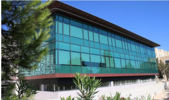
Figure 3: Educational/Office Building used to test the methodology (Source: Author)
