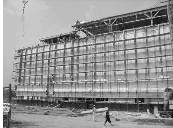
a. Detail from the installation of the envelope walls on the Southern facade
