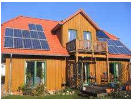
Figure 4. Photovoltaic systems (Etem 2007)
