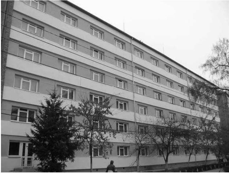
a. South facade rehabilitated – general view
