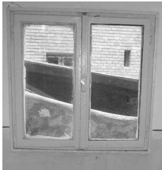
d. Situation of the exterior carpentry
