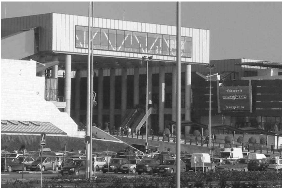
Figure 6. General view of the main entrance of "Iulius Mall" Centre of Timișoara
