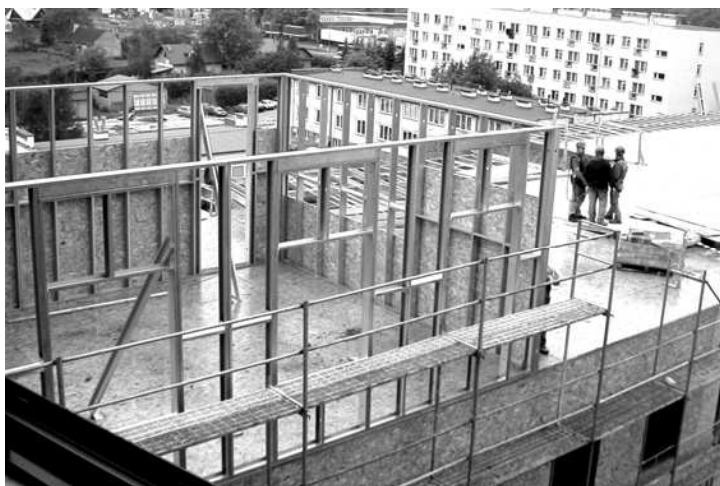
Figure 1. SUNDAY System under construction
