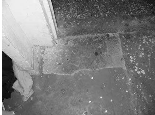
b. Degradation of the linoleum floors
