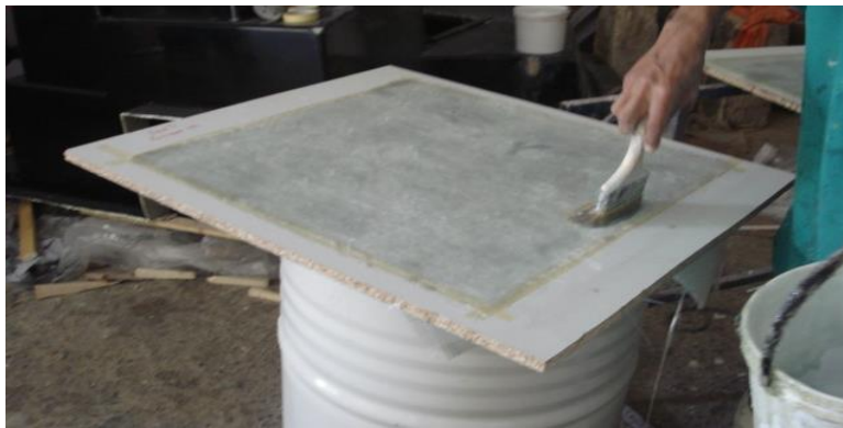
Wetting the reinforcement fabric with resin
