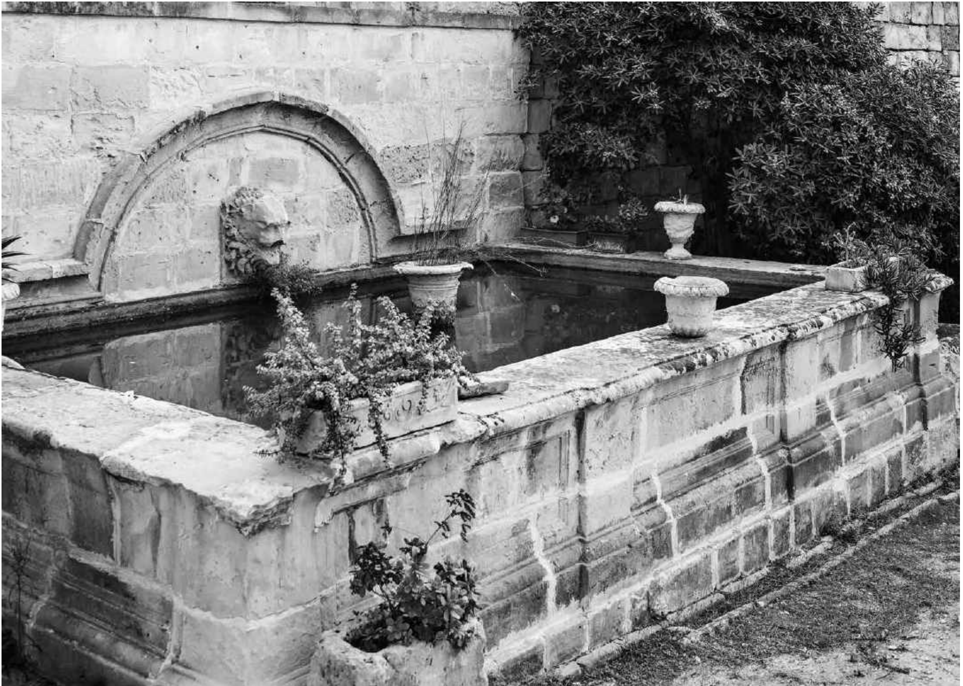
Fig. 62. Stone water reservoir with lion-head gargoyle framed within arch-moulding
