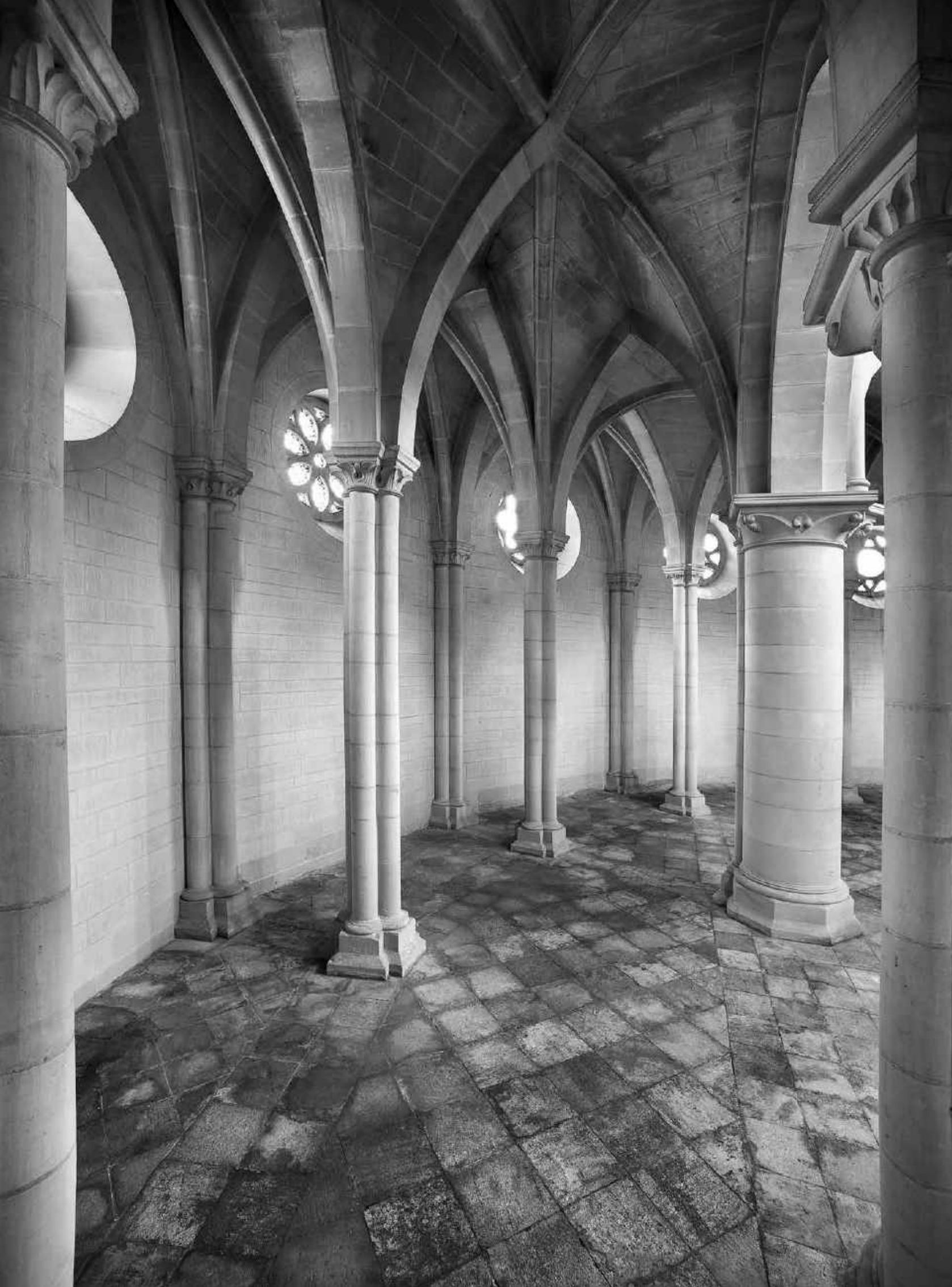
Fig. 122. Vaulting of ambulatory
