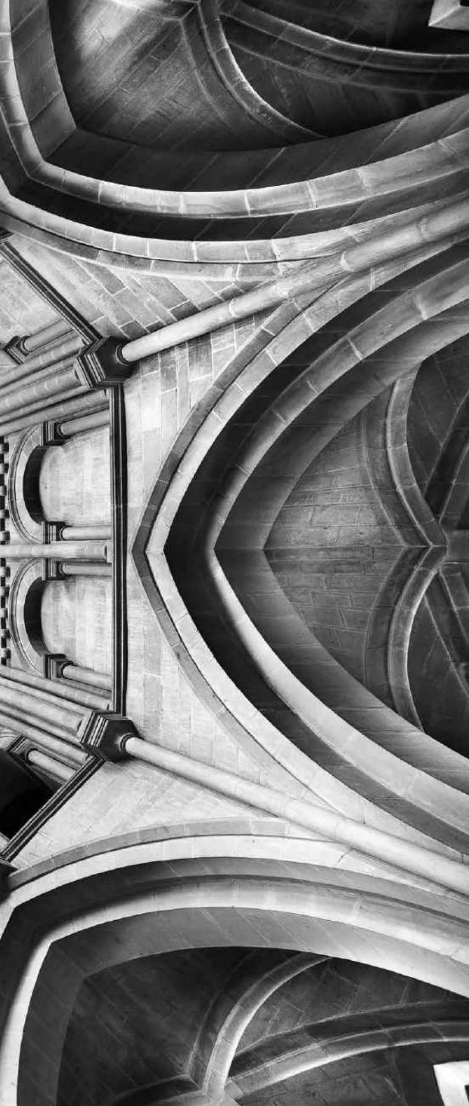
Fig. 121. Internal view of dome and crossing
