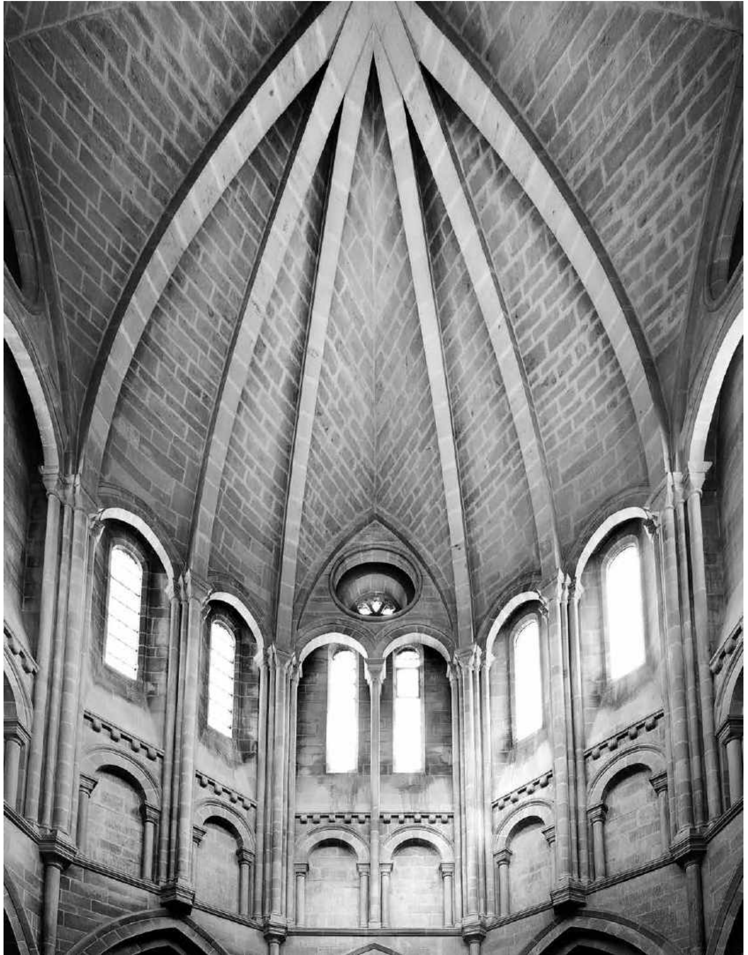
Fig. 120. Internal view of dome
